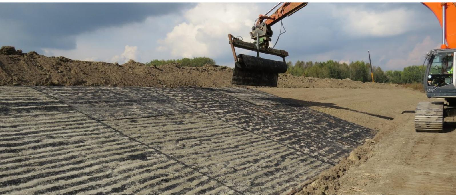
MATELAS ANTI-ÉROSION FLEXIBLE COMPOSÉ DE GÉOTEXTILE, DE GRAVIER ET DE BITUMES
