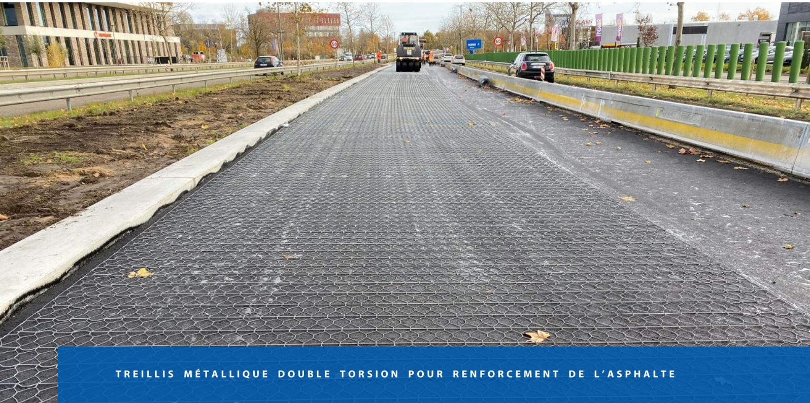
TREILLIS MÉTALLIQUE DOUBLE TORSION POUR RENFORCEMENT DE L'ASPHALTE
