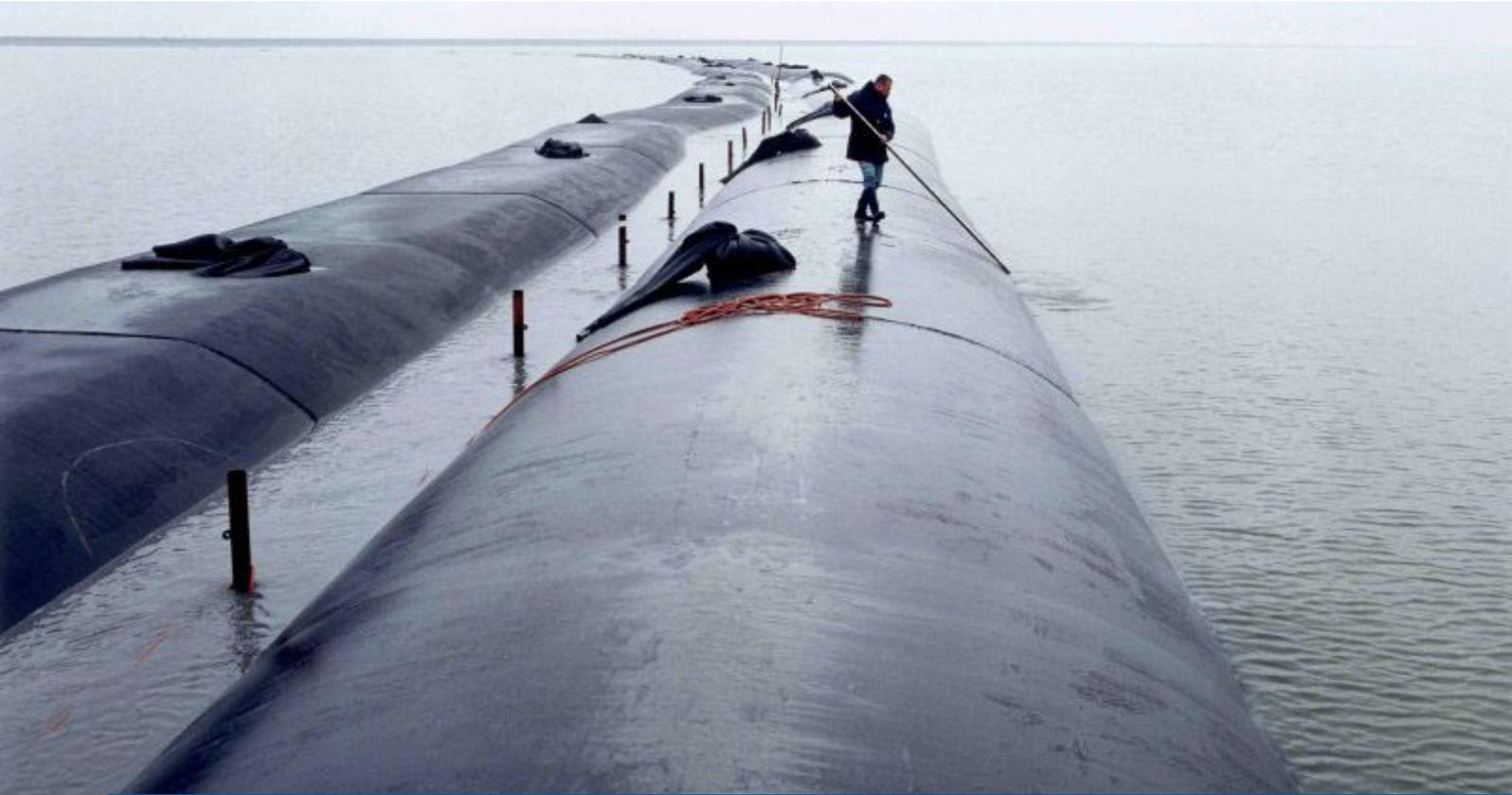
CONSTRUIRE AVEC DES TUBES PERMÉABLES EN GÉOTEXTILE, REMPLIS DE SABLE
