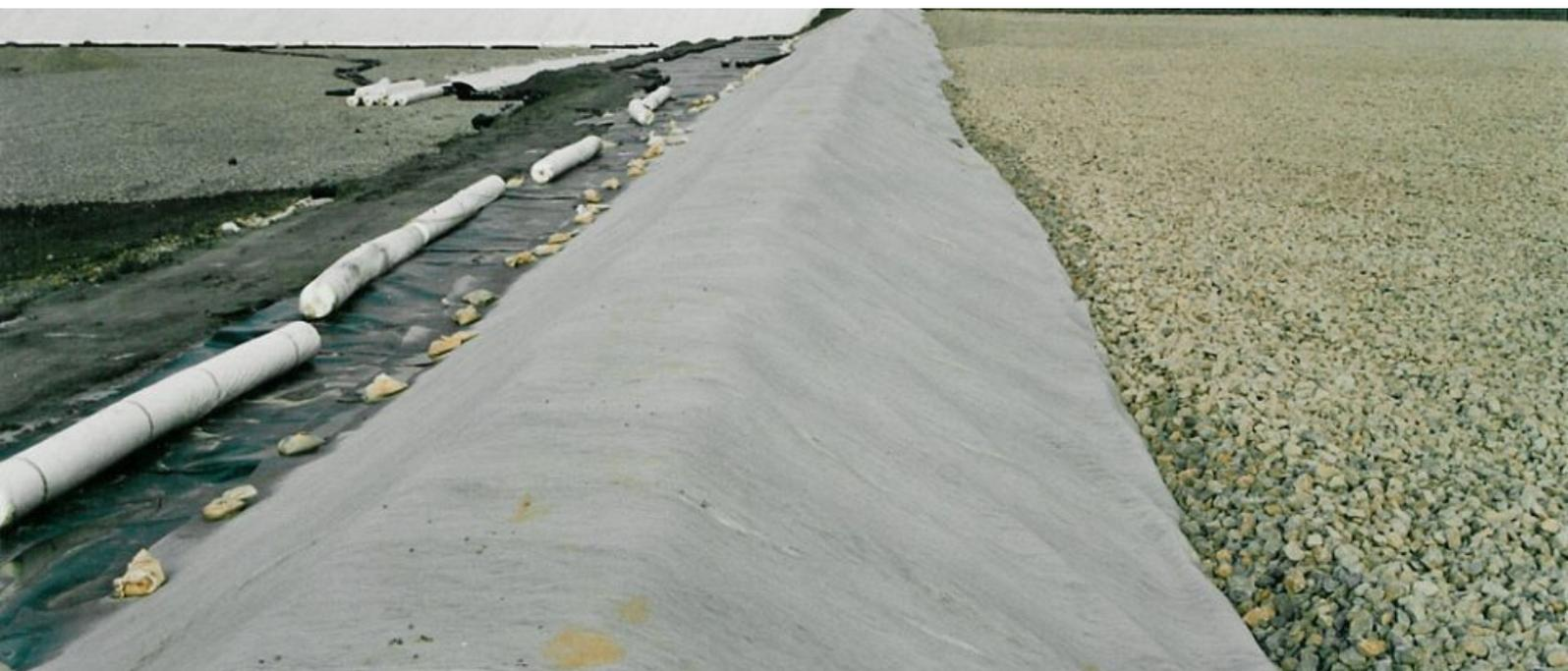
GÉOSPACEURS DE DRAINAGE EN MONOFILAMENTS
