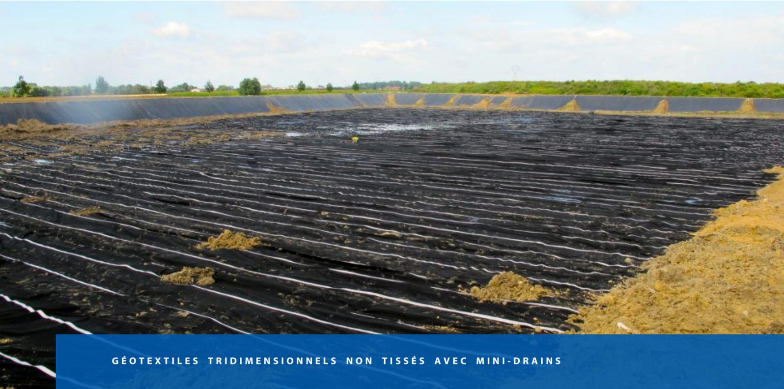
GÉOTEXTILES TRIDIMENSIONNELS NON TISSÉS AVEC MINI-DRAINS
