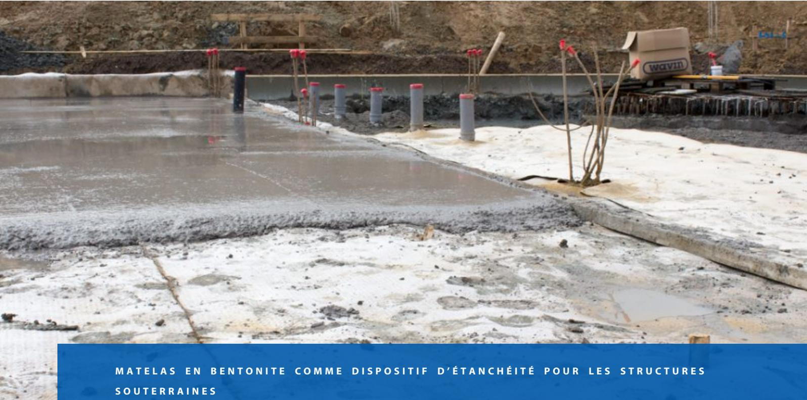
MATELAS EN BENTONITE COMME DISPOSITIF D'ÉTANCHÉITÉ POUR LES STRUCTURES SOUTERRAINES
